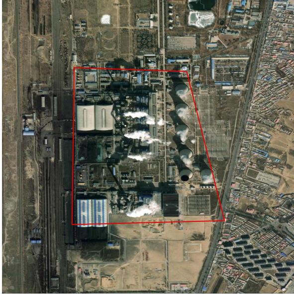
(a) Dalate Steam Plant (Coal) in Dalate, China
