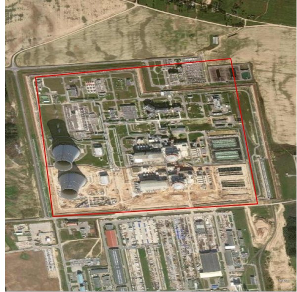
(b) Ostrovets Nuclear Power Plant in Astravyets, Belarus
